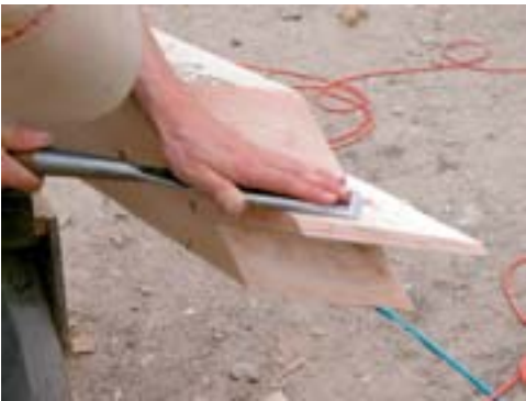
Above: The finished frame in the Kauai 2002 workshop. Posts were scribe fit to stones. Below: Student paring a jack rafter foot in the May 2003 Advanced Timber Framing workshop at FMSTB in Maine.
