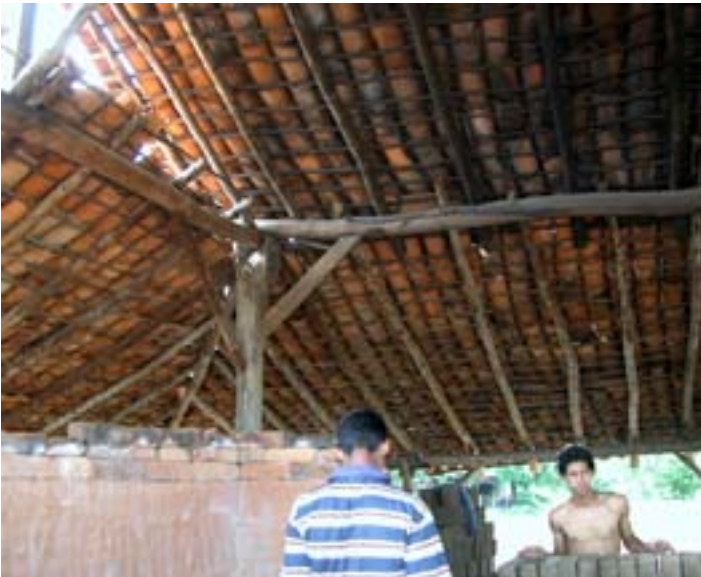
Typical framing of the work sheds covering a kiln. The system is a combination of joinery and lashing, with the tejas laid on top with no fasteners.
