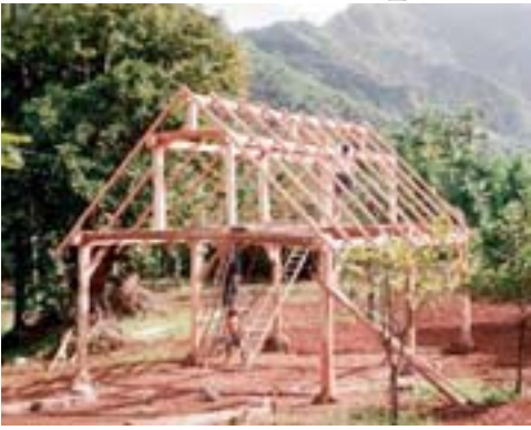
Above: The finished frame in the Kauai 2002 workshop. Posts were scribe fit to stones. Below: Student paring a jack rafter foot in the May 2003 Advanced Timber Framing workshop at FMSTB in Maine.
